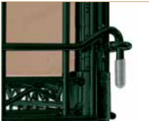
Protective cover on exposed wire ends.
